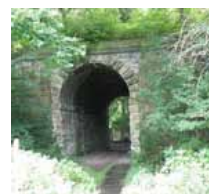
17. The railway tunnel.
